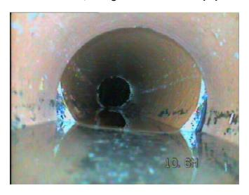
The cause of the blockage was found to be a broken pipe joint, probably due to an adjacent excavation made for the footings of a garden wall done six months earlier, there was no evidence of tree roots in the pipe. Root cutting could have smashed this broken joint further and relining would have done nothing to remedy this offset joint and may have made the problem worse. We were on site for a total of two hours.
